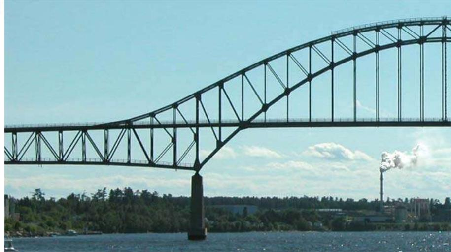
Look at the shapes in the bridge. The beams that form the triangular structures are called trusses. These are very useful in engineering and architecture, because they add strength and stability to structures such as bridges and buildings.
